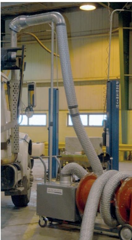
Eliminator Hose Reel Model connected to truck using extended vertical mast
