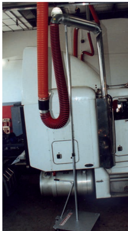
Basic Base Plate Model Eliminator for Truck Application, attached to Overhead Exhaust System
