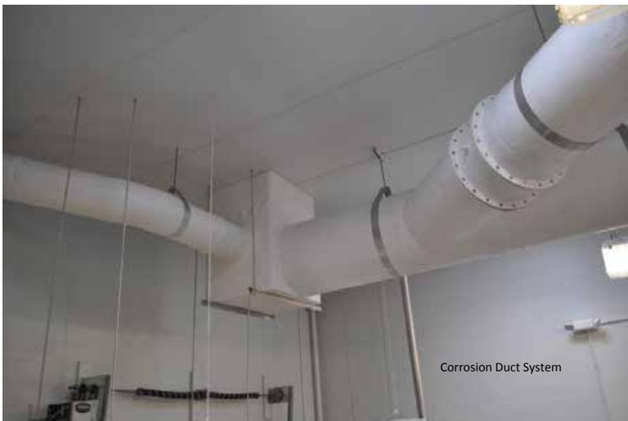
Corrosion Duct System
